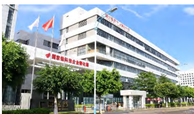
"WePure" Headquarter located in Guangdong
